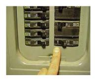
Check circuit breaker to make sure its not tripped Reset if tripped
