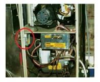
Most furnaces have a blower door safety switch that shuts off furnace Make sure blower door is firmly in place
