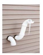
If your furnace is newer and vents out with PVC: Check to make sure venting is not blocked by leaves of ice if cold outside -remove obstructions and see if unit will start
