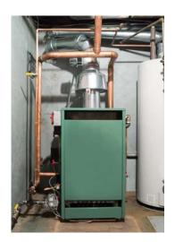
If you have a hot water boiler: Check the pilot light if your unit has a pilot If pilot out re-light according to instructions on unit If pilot will not stay lit or you smell gas shut gas control off and call
